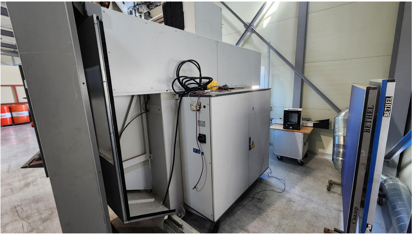
Equipment Detail - View 6
